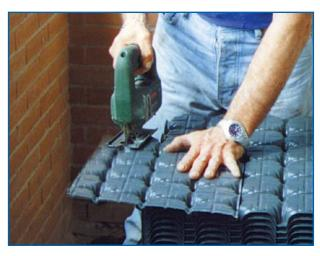
The **MINIMODULO** can be cut with standard tools in proximity of kerbs or wells.
