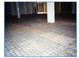
The **MINIMODULO** makes natural or forced ventilation possible over the whole of a surface with **RADON** gas dispersion.
