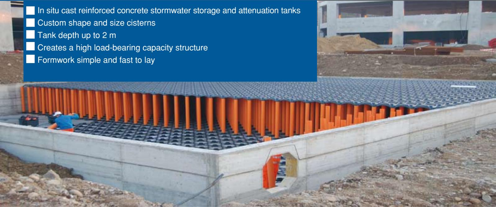
**ELEVETOR® TANK** is an application of **Geoplast's ELEVETOR®** system. The forms are placed after the creation of the tank foundation, floor and walls, including the water inlets and outlets. All the elements of system are made of plastic material that does not degrade in water.
